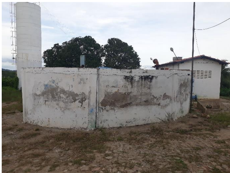
FIGURA 24 - RESERVATORIO SEMI ENTERRADO 45M 3
